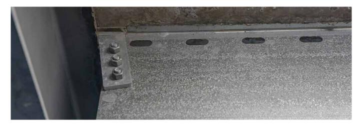
The durability of a galvanised coating is dependent on the thickness of the zinc coating, the general environment and the level of maintenance carried out over the life of the product. Consideration must be given to these factors when specifying SPEEDFLOOR® to determine the longevity of the structural solution. Further clarification of protective coatings and corrosivity zones should be sought from AS/NZS2312:2002 and HERA Report R4 -133:2005.
